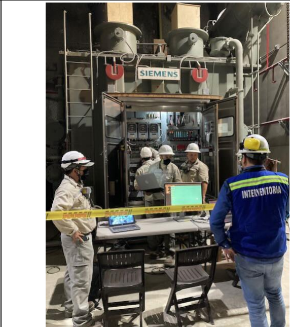
Photo 69: Assembly work in transformer cavern
