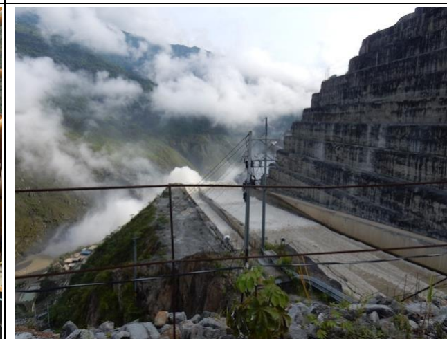
Photo 42: Spillway from dam crest
