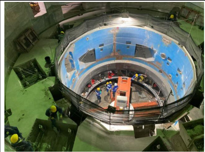
Photo 71: Assembly of generation units
