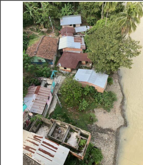
Photo 93: Homes in Puerto Valdivia affected by flood during contingency
