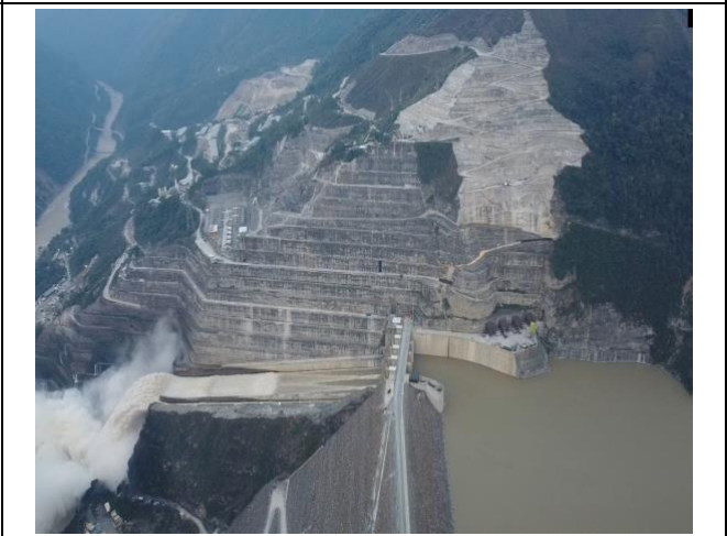
Photo 126: Panoramic view of main works at Ituango project
