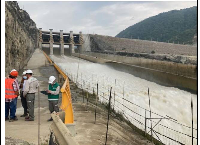
Photo 36: Spillway in operation
