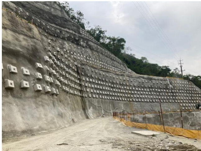
Photo 34: Slope stabilization above dam on right bank
