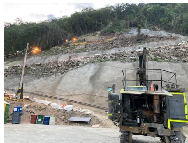
Photo 17: Slope stabilization at 0+900
