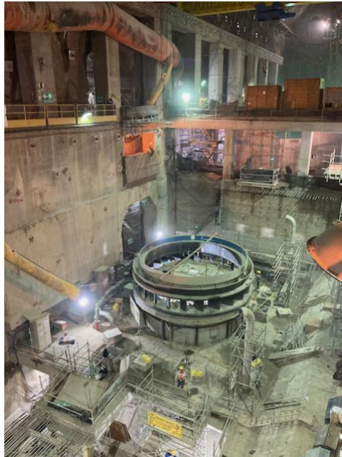
Photo 76: Assembly of generation units
