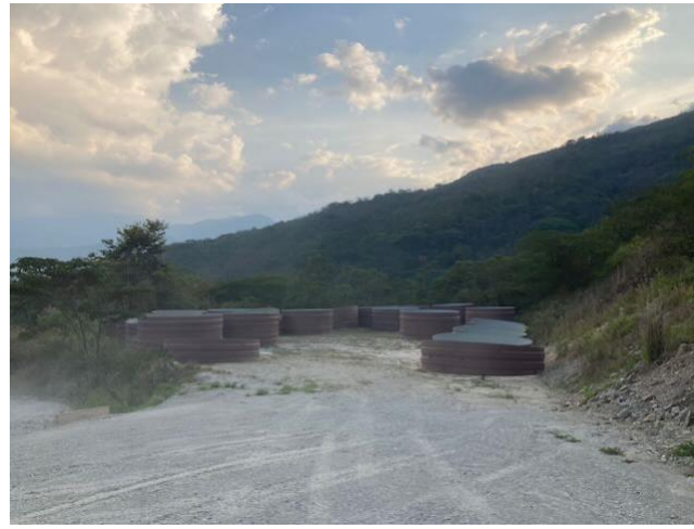
Photo 44: Storage of ferrules to repair intake sections damaged by the contingency, on left bank
