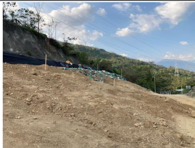
Photo 29: Project landfill in the process of closing and covering
