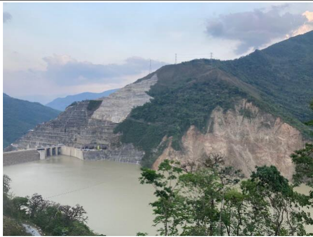
Photo 31: Dam and unstable areas on right bank
