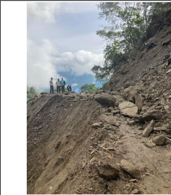
Photo 115: Typical landslide blockage, on road to Toledo rebuilt by EPM as community investment
