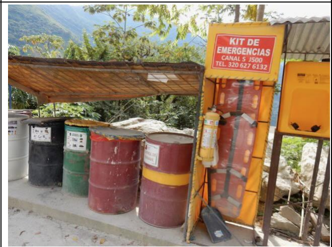
Photo 18: Waste management at slope stabilization site 0+900
