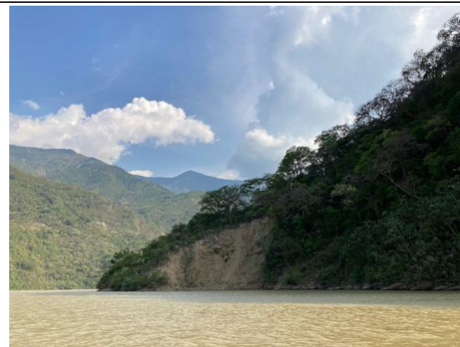
Photo 7: Unstable slope in reservoir 2
