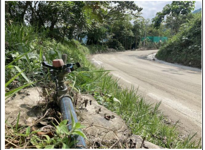
Photo 45: Sprinkler system to suppress dust on main construction roads
